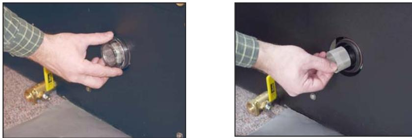
**Figure 6-2. Unscrew See-through Cap (Left Photo); Remove and Inspect Filter (Right Photo)**
