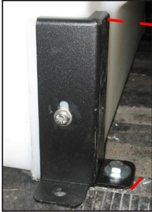
**Figure 2-5. Drill Only 1 Hole for Corner Bracket**
